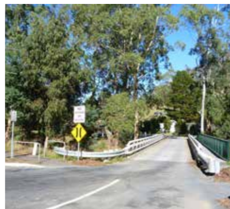
Figure: 2.5.2 The bridge between Broome Road and Whittlesea - Yea Road
