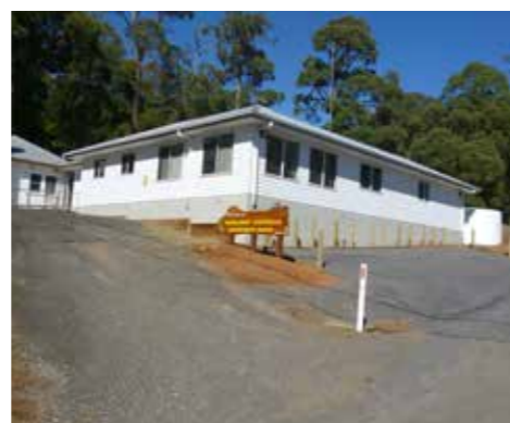
Figure 2.1.1 Toolangi Castella Community House on Toolangi Tennis Reserve
