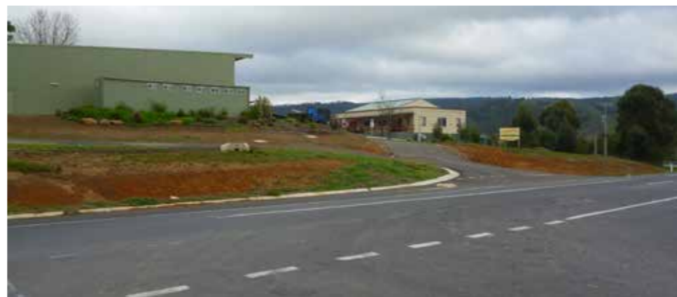
Figure: 2.6.3 View looking south from Broadford - Flowerdale Road, across the Whittlesea - Yea Road toward the Flowerdale Community Hall
