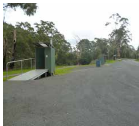
Figure: 2.5.3 The bus stop and toilet on the Whittlesea - Yea Road at Flowerdale Central
