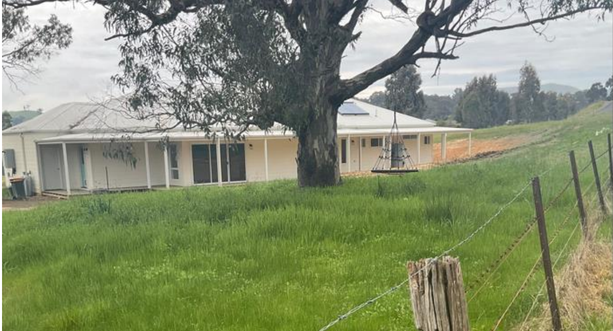
Photograph 1: Existing dwelling at 8 Morgan Drive
