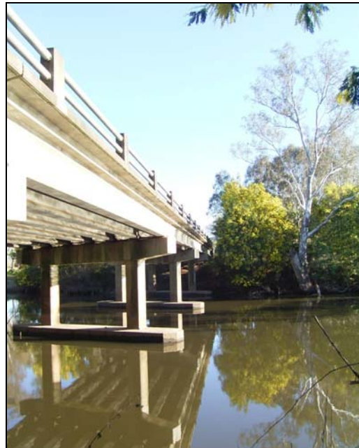
Goulburn River Bridge.
