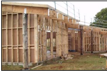
Kinglake District Services Centre under construction.
