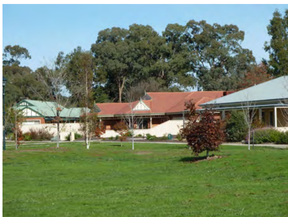
Mulqueeney Lane housing area
