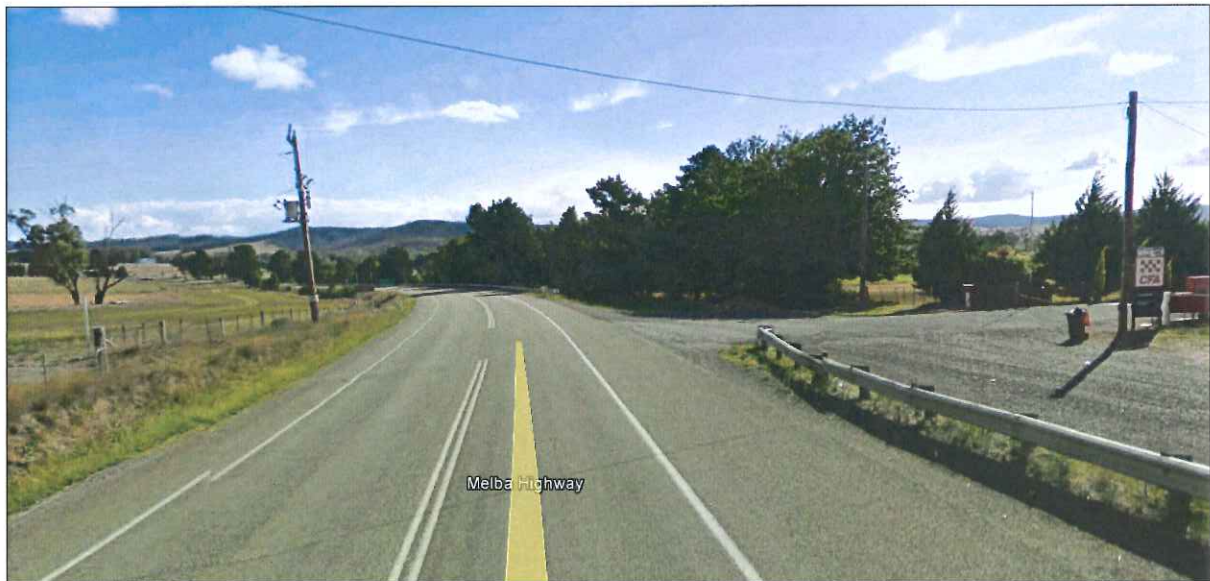
Figure 7 South of the subject site. (Looking North)
