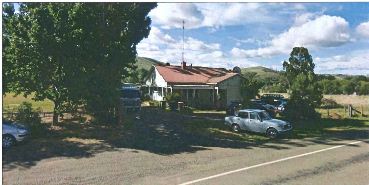
Figure 4 Property to the East of the subject site.
