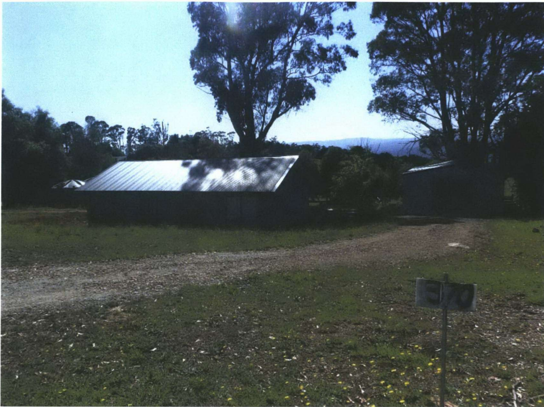
Figure 16: view north of dwelling located on 370 Extons Road
