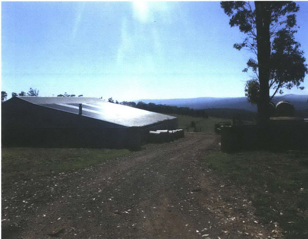
Figure 7: entrance to garage associated with dwelling 2 located in the centre of the frontage
